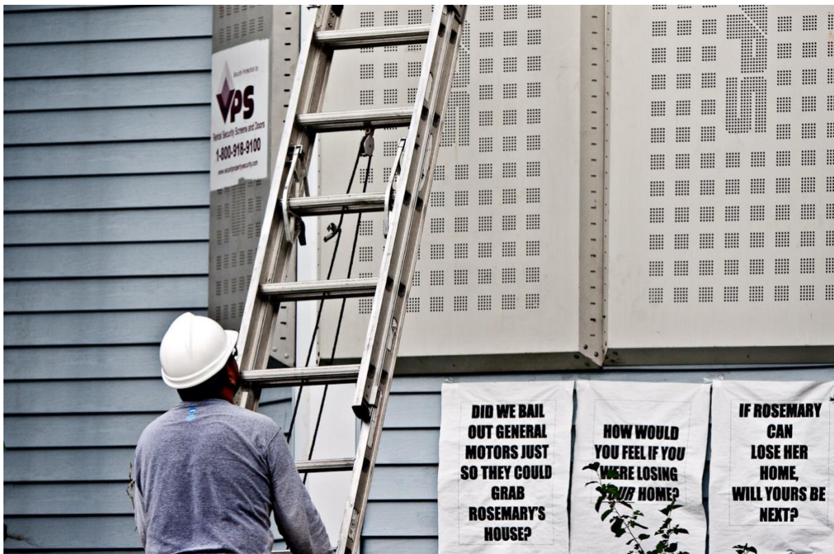
Worker installs security panels over windows after police evict woman from her foreclosed home in South Minneapolis, 2009. (Tony Webster, CC BY 2.0, Wikimedia Commons)
